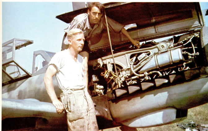
Upper and lower. These two exceptional photographs depict a Bf 109G, White 10, of I./JG 52 being serviced somewhere on the Eastern Front. The lower shot shows particularly good detail of the Daimler-Benz engine and the way the divided cowling panels hinged at the top. Of special interest is the obviously fairly new factory scheme featuring RLM 76 on the upper flying surfaces in conjunction with the same color elsewhere plus liberal blobs of RLM 02, 74, and 75. Even though the yellow rear fuselage band was also fairly new, its pale color is obvious.
